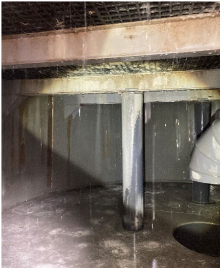
SWTP Degasifier A - Pictures of the interior after the collapsed (2024)
